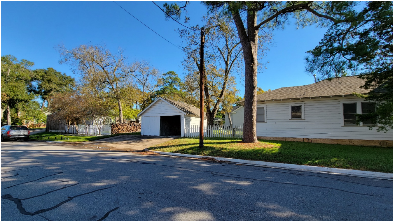
View from directly across subject property. Nonconforming Accessory structure on the NE corner lot of Academy & Hosea Streets.
